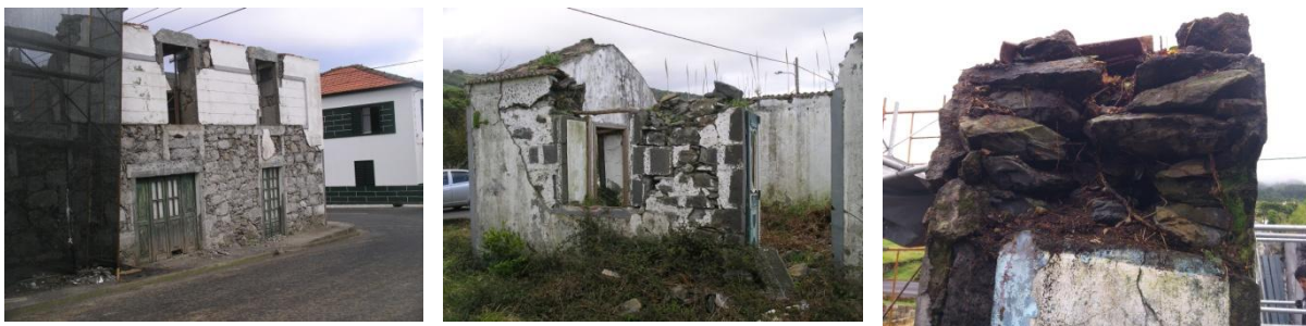
Fig. 6: Typical Azorean masonry houses used in the experimental tests
