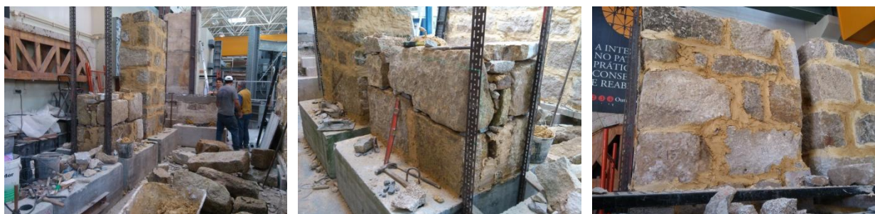
Fig. 16: Construction images of the specimens
